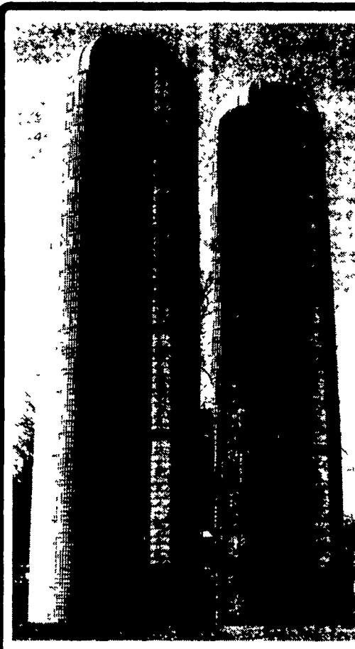
After The surface is reconditioned, and a new, thick, tough surface will protect stored feed
