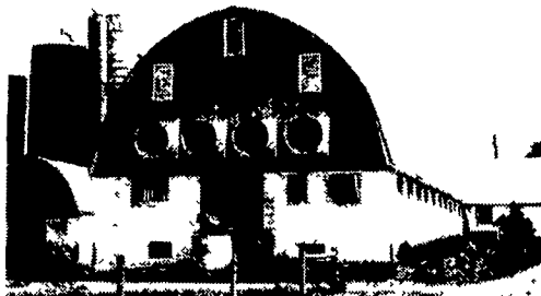
Tie Stall Barn, Myerstown, PA
