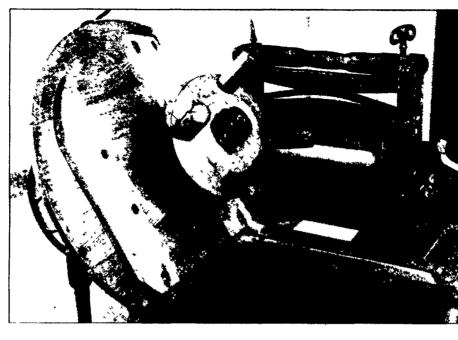
The Pan-American Washer, patented in 1883, employed this central agitator, which operated back and forth. The bottom-mounted agitators of today's washers employ similar back and forth motion. The wringer was made by the American Wringer Company and patented in 1888. The concept of the agitator is one of a very few inventions that have lasted over 100 years. Today washing machines use an agitator only operated from the bottom by electric motor. -Pasto Agricultural Museum, Penn State University.
