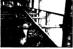
23/8" OD 10 gauge High Tensile Galvanized Steel Tubing Hot Dipped Galvanized Clamp and Mounting Hardware
