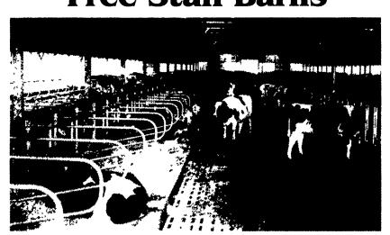
The concrete slat with your animals comfort in mind. A large percentage of openings keep animals clean & dry, waffle slat for better footing. Concrete slats poured with 8,000 PSI concrete, steam cured, for extra strength.
