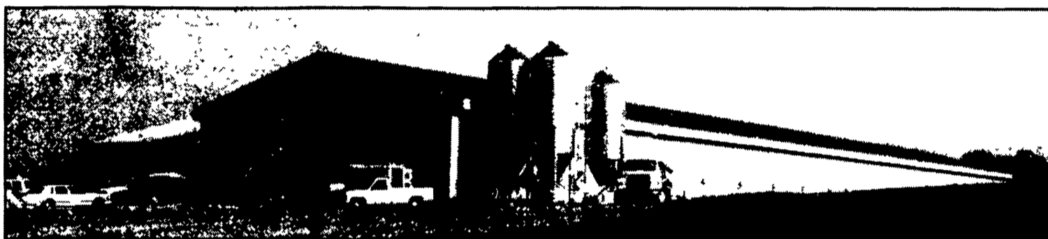
75' x 464' High Rise Layer House with 40'x60' Work Room and Cooler featuring Poured Concrete Walls.
