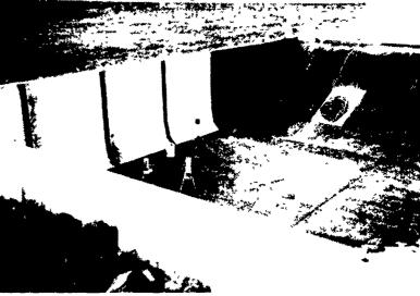
**Precast Walls Sealed With** Welded HDPE LINER **Leak-Proof With Underground Detection Lines.** All Sizes Above Or Inground Sets-Up Quickly.
