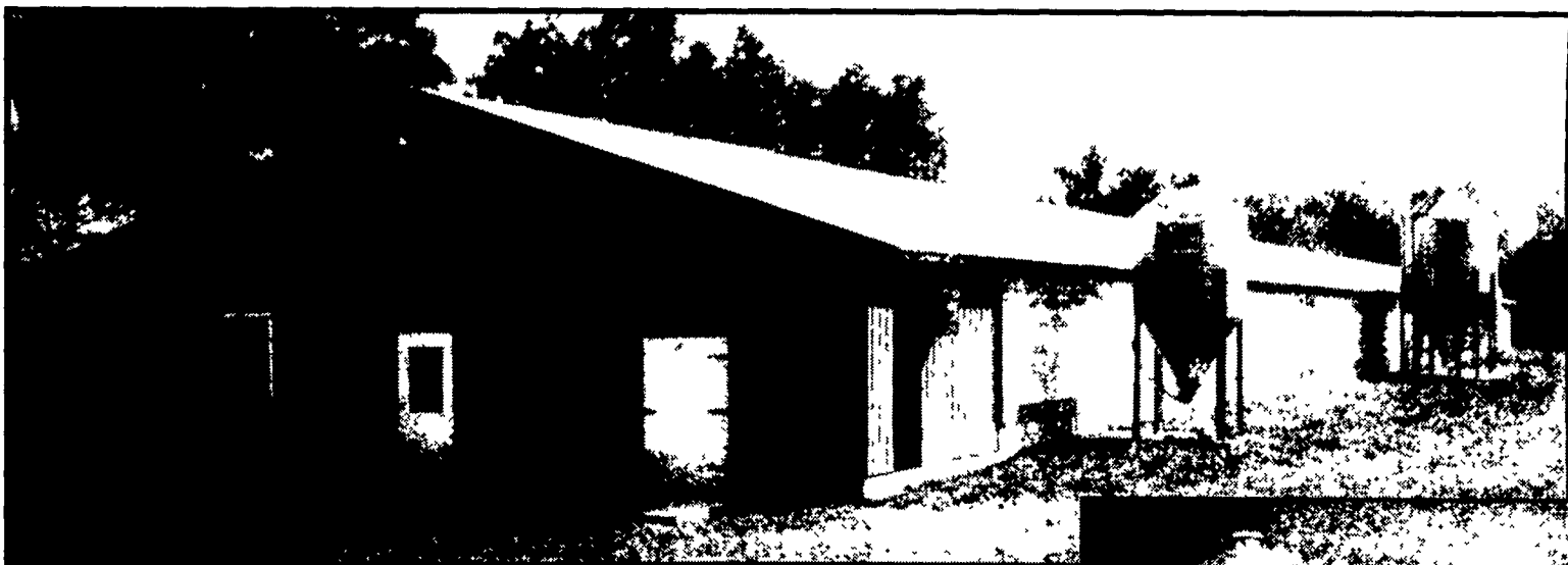
42'x328' curtain sided building constructed by Northeast Agri Systems
