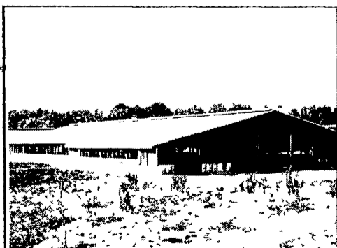
Free Stall Barn Exterior
