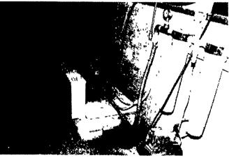
High pressure pump is controlled by temperature and humidity levels. Water is filtered and injected to prevent calcium build ups in lines and nozzles.
