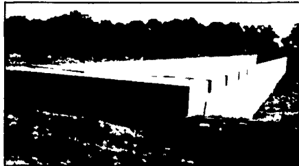
300' Long Manure Pit For Hog Confinement
