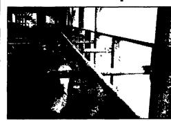
2%" OD 10 gauge High Tensile Galvanized Steel Tubing Hot Dipped Galvanized Clamp and Mounting Hardware
