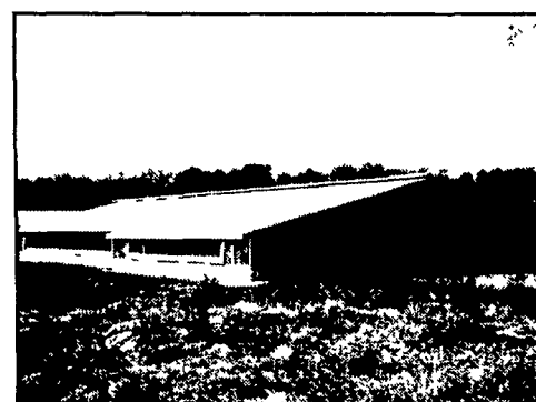
Free Stall Barn Exterior
