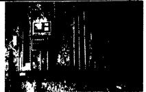
SIMPLE, VERSATILE, and AFFORDABLE SUPER-Selector" Chore-Time\* Ventilation Control is a user-friendly 12stage microprocessor control designed to efficiently work with nearly all ventilation methods - natural, negative satic pressure, and tunnel. Easy to operate, this control features two heat and 10 cooling stages. The SUPER-Selector is easy to set up and adjust to fine tune for your building's specific ventilation requirements.
