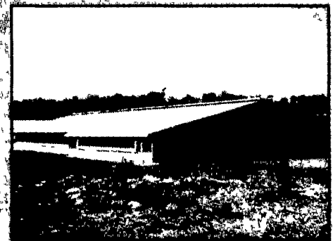
Free Stall Barn Exterior
