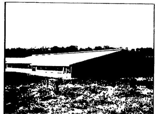
Free Stall Barn Exterior
