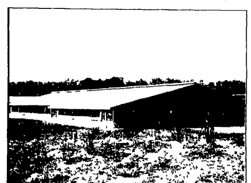
Free Stall Barn Exterior
