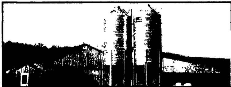
New tunnel ventilated broiler house featuring Chore-Time C2 feeders, Chore-Time PMT automatic tunnel controls and Hired Hand System 2000 automatic tunnel control.
