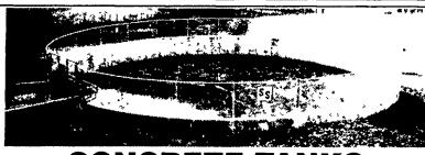
Poured In Place Or Precast Up to 140' Diameter Or Rectangle, Even or Uneven Back Fill We Can Custom Design Your System.
