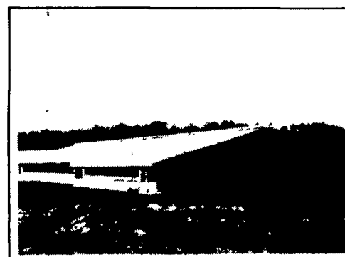
Free Stall Barn Exterior
