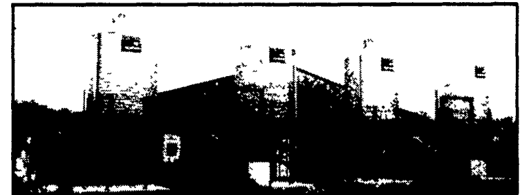
3,200 capacity "side by side" tunnel ventilated hog finisher featuring Chore-Time bins and augers and Staco stainless feeders.
