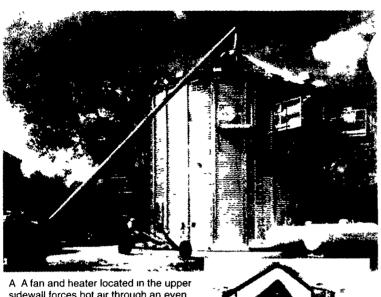
sidewall forces hot air through an even column of wet grain above
