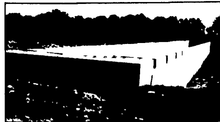
300' Long Manure Pit For Hog Confinement
