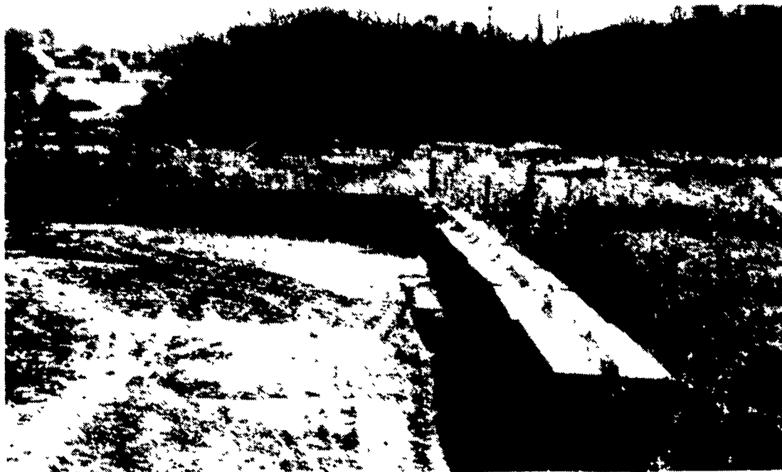
Runoff water from the rest of the barnyard is directed through a picket fence to filter solids and then to a fenced off grass filter area to treat liquids.
