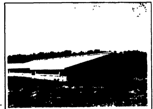
Free Stall Barn Exterior
