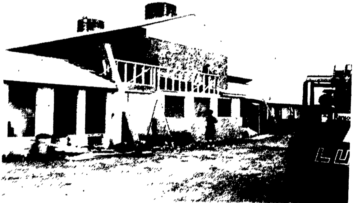
The Mertz family is grateful to the many volunteers who helped rebuild and cleanup after tornado damage.
