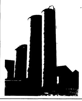
With A 6" Thick Wall, Ambient **Temperatures And Sun Have Limiting Effect** On Interior Temperature Resulting In **Better Quality** Corn.
