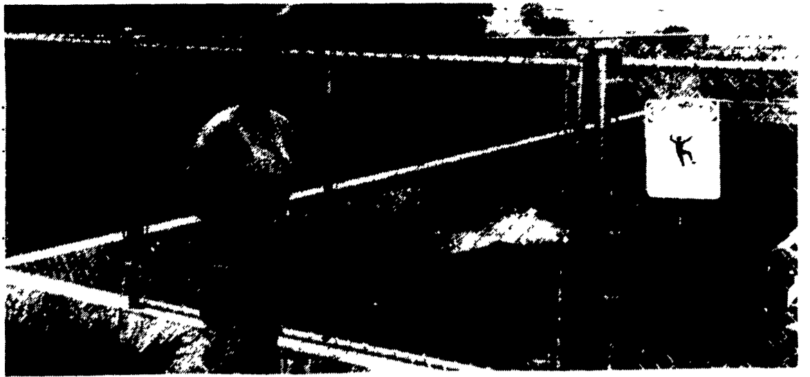
There are similar projects that have already been installed on local farms. One Marion Township farm completed construction on this concrete-lined manure impoundment structure, installed in the spring of last year, inspected by Kim Fies of the Berks conservation district. The poured wall storage structure contains 8-inch thick by 8-foot long forms arranged in a rectangular shape, to a depth of about 8 feet.
