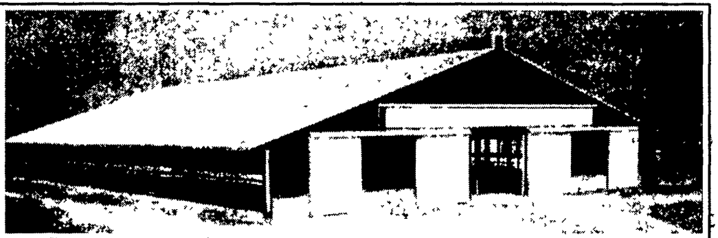
Concrete Slatted Free Stall Barn
