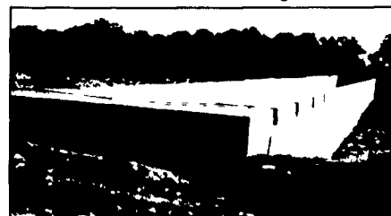
300' Long Manure Pit For Hog Confinement
