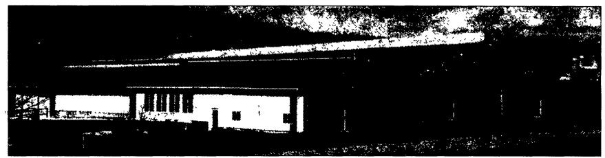
300 cow free stall barn and milking center with sort area for breeding & health checks. Designed & built by Triple H Construction, Ephrata, PA. Featuring: Cow Mattresses by North Brook; Paul B. Zimmerman Fencing & Gates; Berg-Bennett Free Stalls; Kipe Dump Waterers; Rigidply Rafters; Groffdale Poured Concrete Walls; Keystone Waffle Slats; and Rubber Padding at Feed Area.
