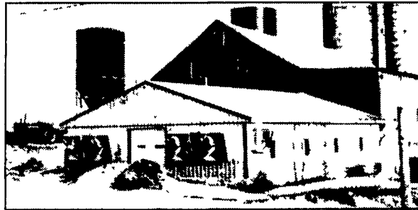
Mr. and Mrs. Mike Stoltzfus, Clearville, Pa. Tie Stall Barn Addition.
