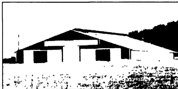
Hillcrest Saylor's Dairy Farms, Rockwood, Pa. 200 Cow Freestall Barn
