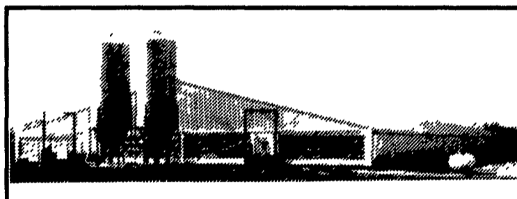
3,200 capacity "side by side" tunnel ventilated hog finisher featuring Chore-Time bins and augers and Aerotech fans and controls.
