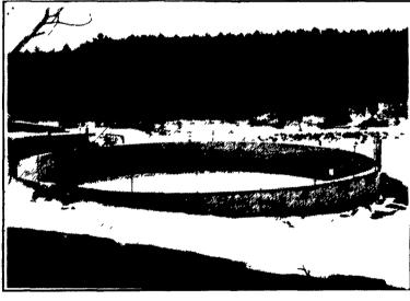
Partial In-Ground Tank Featuring Commercial Chain Link Fence (5' High - NRCS Approved)
