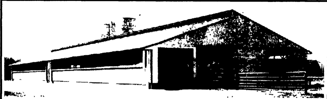
Concrete Slatted Free Stall Barn
