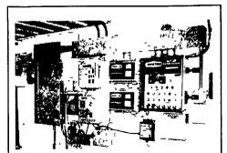
SIMPLE, VERSATILE, and AFFORDABLE Chore-Time® SUPER-Selector PNT Ventilation Control is a userfriendly 12-stage microprocessor control designed to efficiently work with nearly all ventilation methods natural, negative satic pressure, and tunnel Easy to operate, this control features two heat and 10 cooling stages. The SUPER-Selector is easy to set up and adjust to fine tune for your buildings specific
