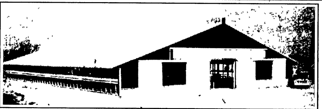
Concrete Slatted Free Stall Barn
