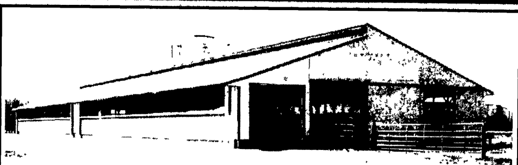
Concrete Slatted Free Stall Barn
