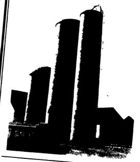
With A 6" Thick Wall, Ambient **Temperatures** And Sun Have Limiting Effect On Interior **Temperature** Resulting In **Better Quality** Corn.
