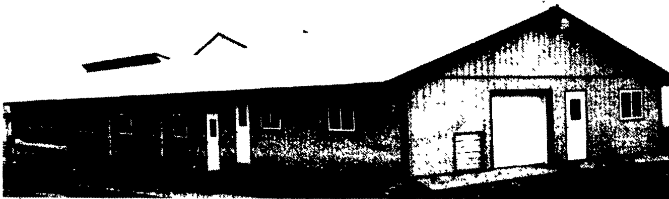
All New Milking Center & Holding Area with Curtain Sidewalls and Glasbord Walls.
