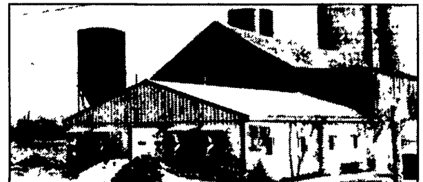
Mr. and Mrs. Mike Stoltzfus, Clearville, Pa. Tie Stall Barn Addition.
