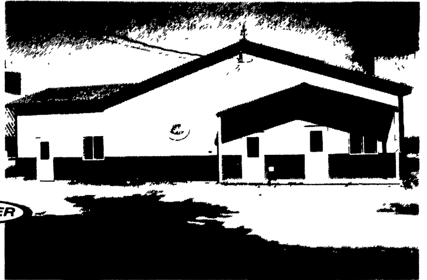
43'x159' Milking Center & Holding Area.
