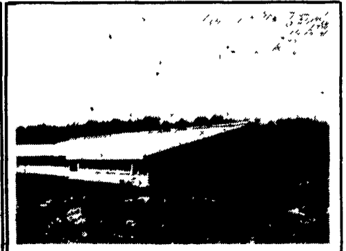
Free Stall Barn Exterior
