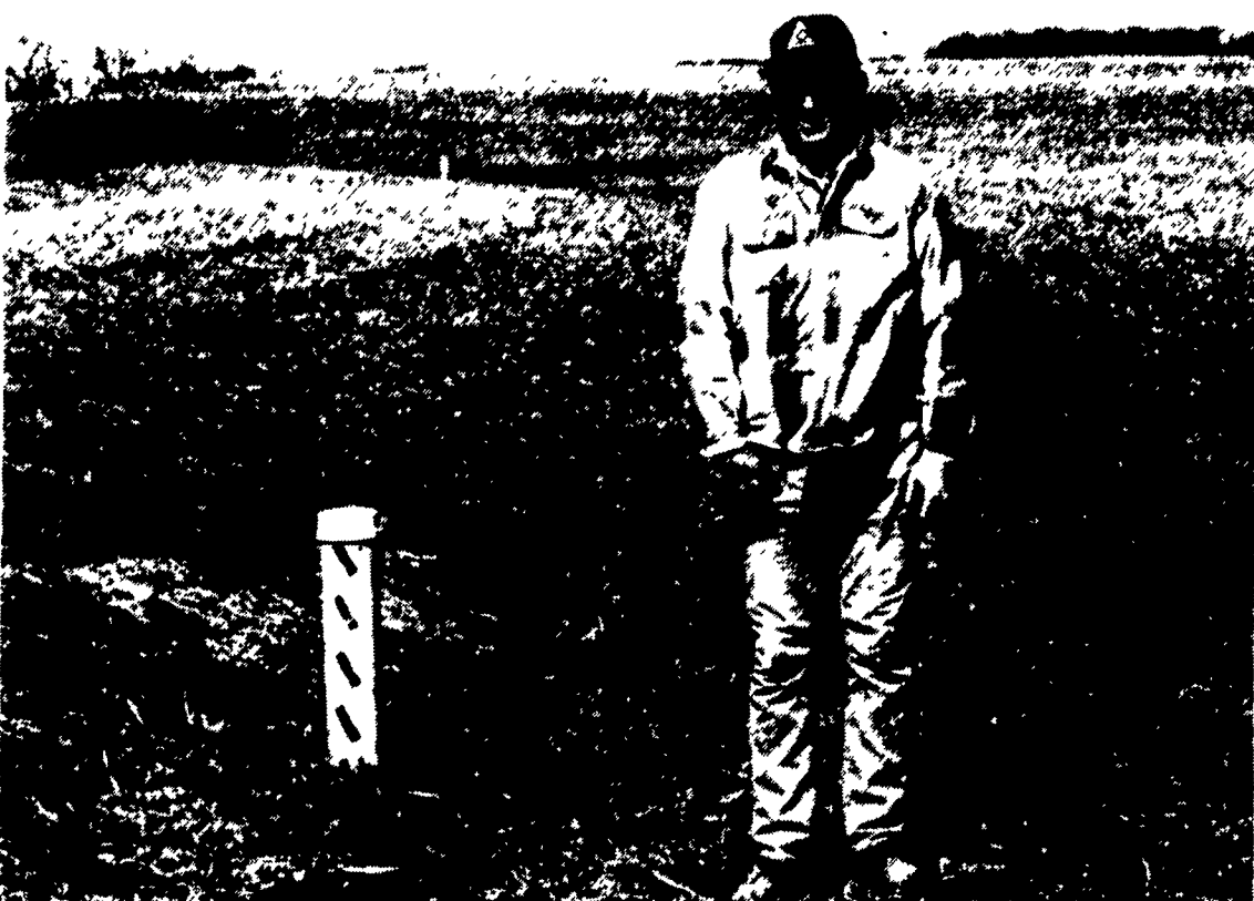
The terraces were the real key to stopping the flooding and erosion. But it's "something that's going to have to be maintained," said Moyer. Moyer shows the pipe inlets from one terrace.
