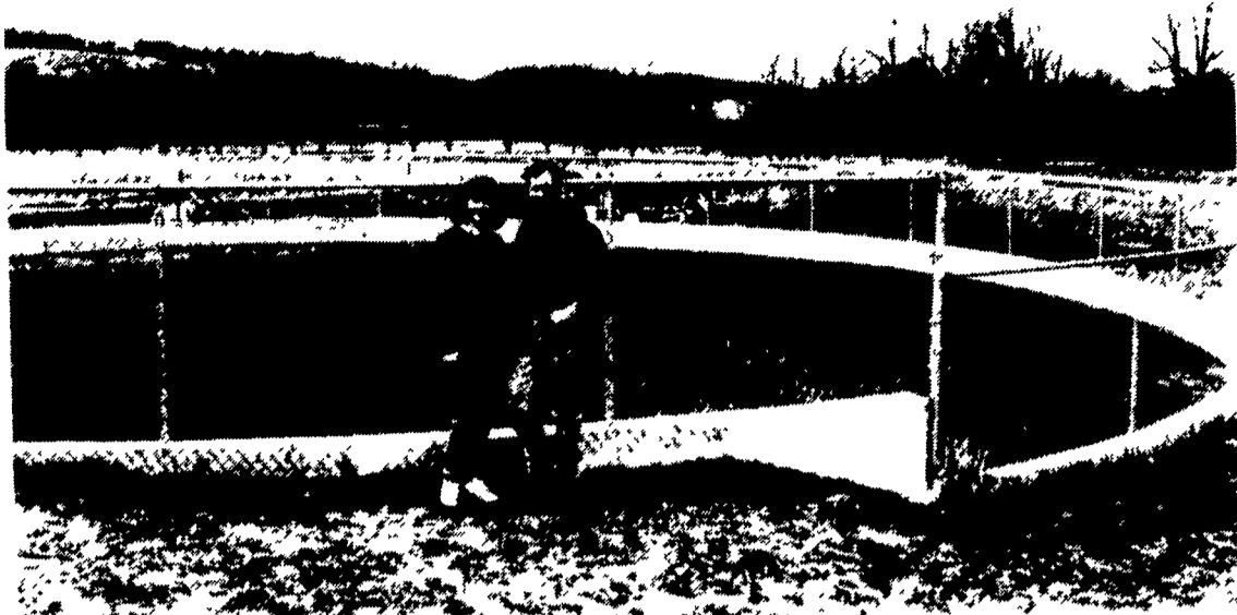
In 1992, the Umbles signed a Chesapeake Bay contract to cost-share the construction of a eight- by 60-foot circular concrete manure storage structure.
