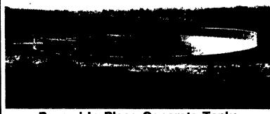
**Poured In Place Concrete Tanks** SCS Approved 6', 8', 10', 12', 14', 16' Depths Thru 140' Diameter **Even And Uneven Backfill Designs Commercial Chain Link Fence**
