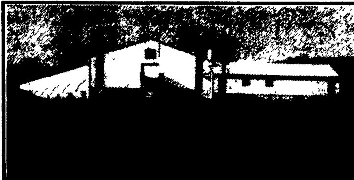
54'-8" x 612' High rise building with 36' x 60' egg packing and cooler room. Building features brown-out Inlet hood and treated lumber decks at bird load out doors.
