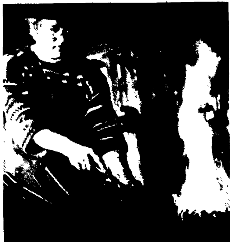
Welding within the forge takes a practiced eye. Flux is added to help fuse two pieces of iron.
