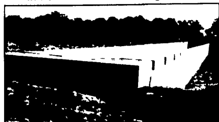
300' Long Manure Pit For Hog Confinement
