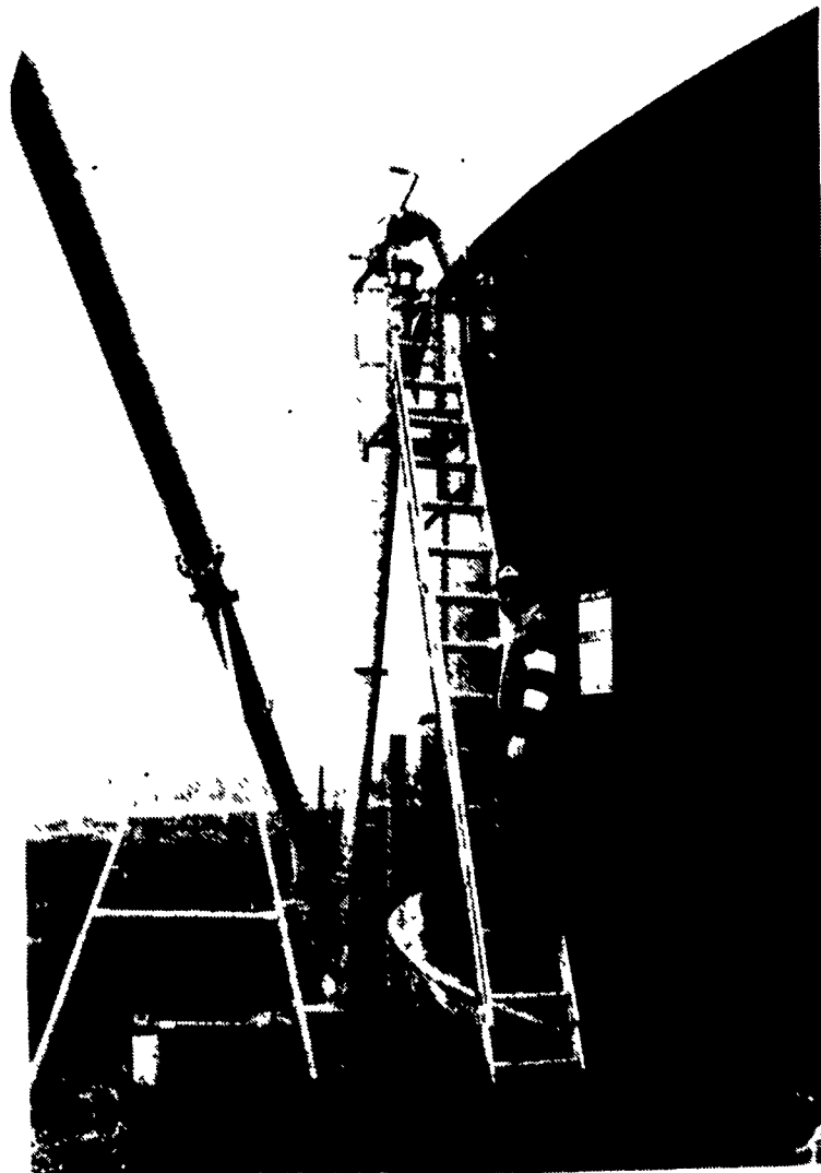
As part of the conservation plan, initiated in May 1992, a 316,000-gallon manure storage tank was installed in July 1992. The tank is emptied twice a year, or every six to seven months. It was put up with a cost-share program available through the Chester County Conservation District.
